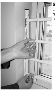
Step 1 Locate all emergency release buttons indicated by labels.
